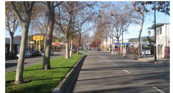
In contrast to San Pablo Avenue in Albany, the Berkeley segment of San Pablo is characterized by wide, green, well-maintained medians with high canopy trees.
