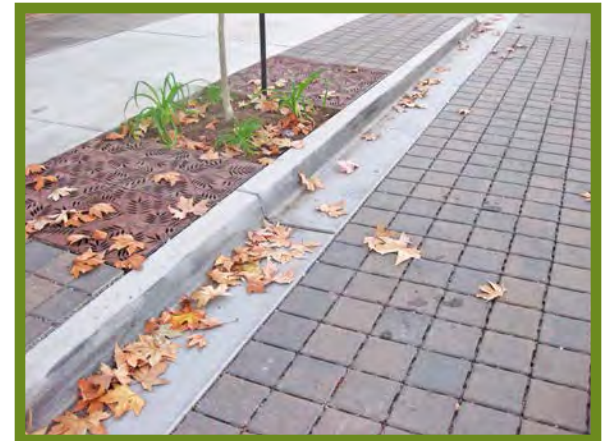
Tree grates protect trees and create a clean, accessible ground plane. Larger openings benefit tree health by maximizing non-compacted soils. Subsurface treatments to improve soil volume for tree roots should also be studied for San Pablo Avenue. (Castro Valley, CA)
