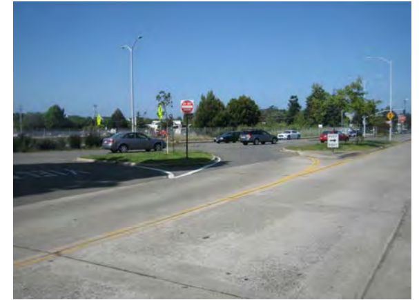
Existing intersection of Buchanan Street and Marin Avenue.
