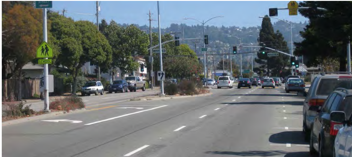
On Buchanan Street, the lack of a mature tree canopy for scale contributes to high speed conditions. While the community effort to install the adapted coastal scrub planting improvements several years ago is applauded, the median requires ongoing maintenance in order to keep sightlines clear. Future plantings should address sightlines to crosswalks and crossing vehicles.
