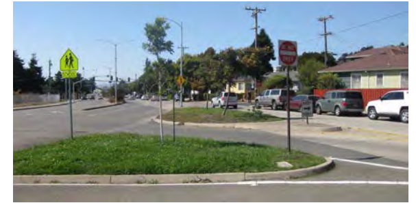
The configuration of the skewed Buchanan Street and Marin Avenue intersection creates a series of underutilized, "leftover" median spaces. The configuration also prevents pedestrians from safely accessing the City Hall sidewalk on Marin Avenue from the north side of Buchanan Street.
