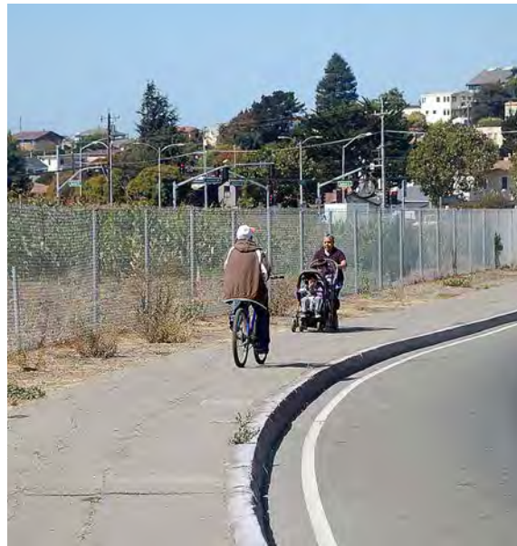
Cracked and broken sidewalk on Buchanan Street, which is also narrow with no buffer from the vehicular lanes.
