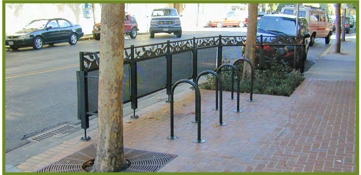
U-shaped bicycle racks placed on a curb extension to avoid conflicting with sidewalk zone.
