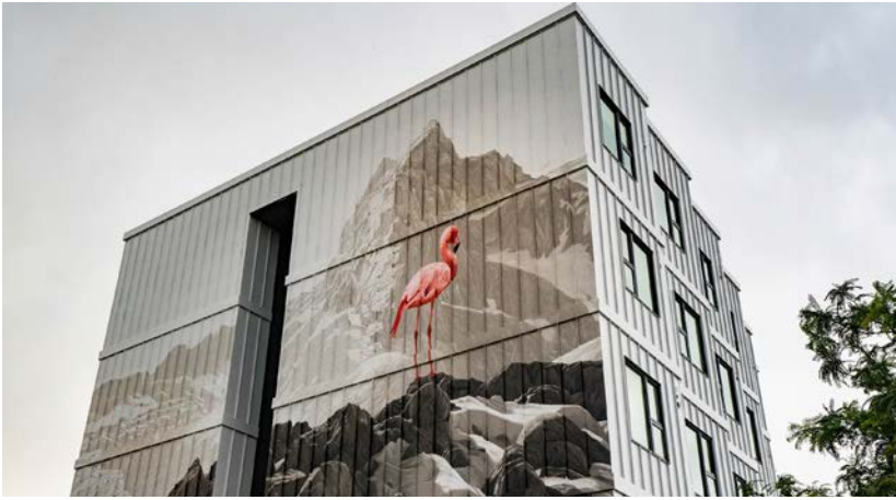
Murals on side facades at the zero lot line should be enhanced with public art. (The Exchange, Salt Lake City, UT - Francisco Kjolseth | The Salt Lake Tribune)
