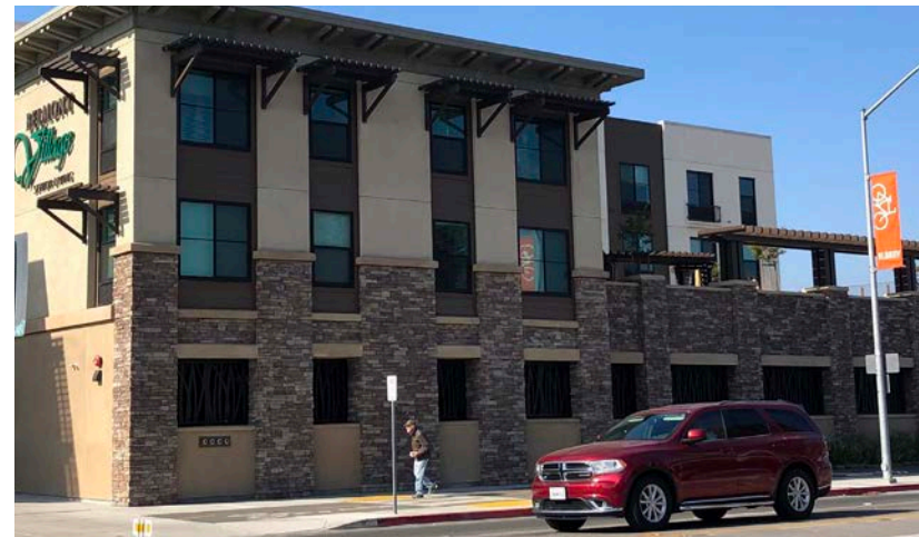
The ground level of the Belmont Village in Albany is a parking garage which is designed to be integrated with the appearance of the main building. The design includes decorative metal grates that screen the vehicles inside and human scaled, high quality materials at the pedestrian level.
