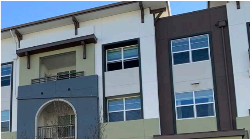
Example of painted vents, gutters, and downspouts.
