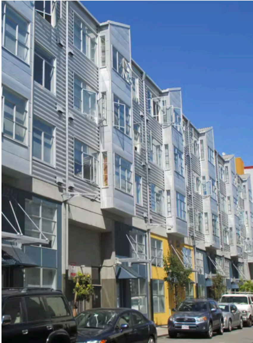
Live/work units on the ground-floor (Adrienne Doyon)
