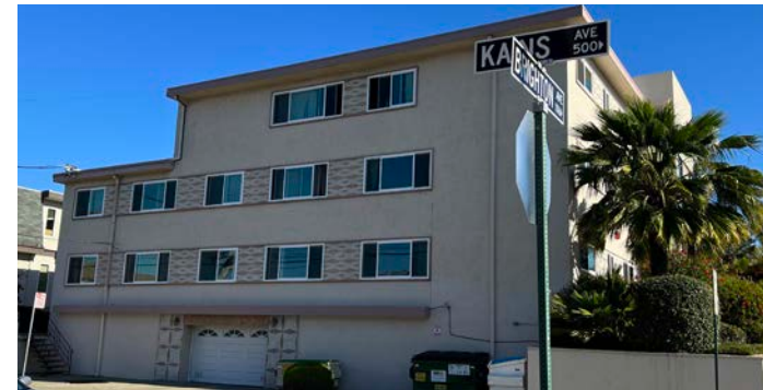
Older 4-story Apartment Building on Kains
