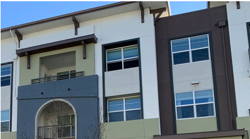
Example of painted vents, gutters, and downspouts.
