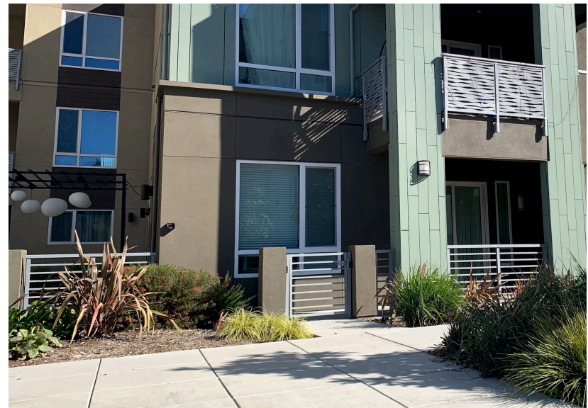
Individual Residential Entries shall provide a transition zone between the public pathway and the entrance to the unit. This can be accomplished with a stoop, porch, or patio.
