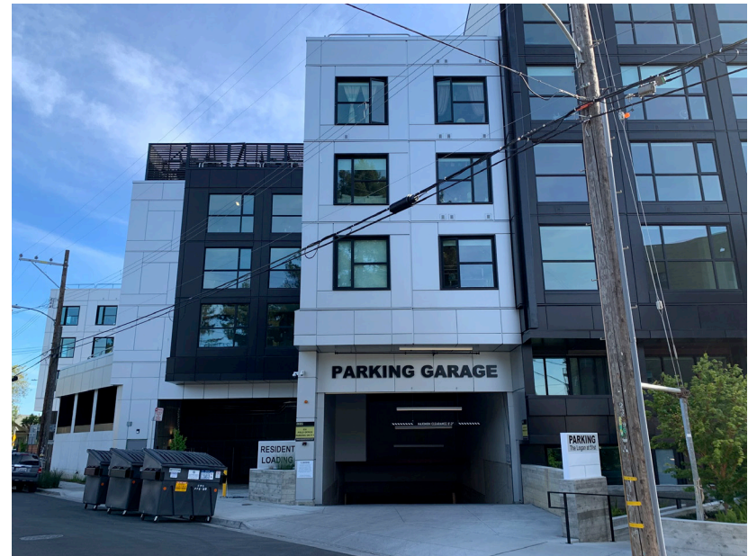
The service area is placed on a side street and is concealed from the street. The refuse containers are out for pickup in this image.
