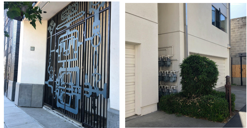
Ideally, utility boxes are screened or hidden behind landscaping or architectural screening.
