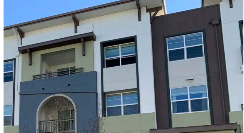
Example of painted vents, gutters, and downspouts.
