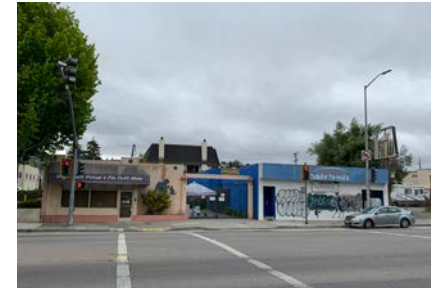
Typical Older One Story Building
