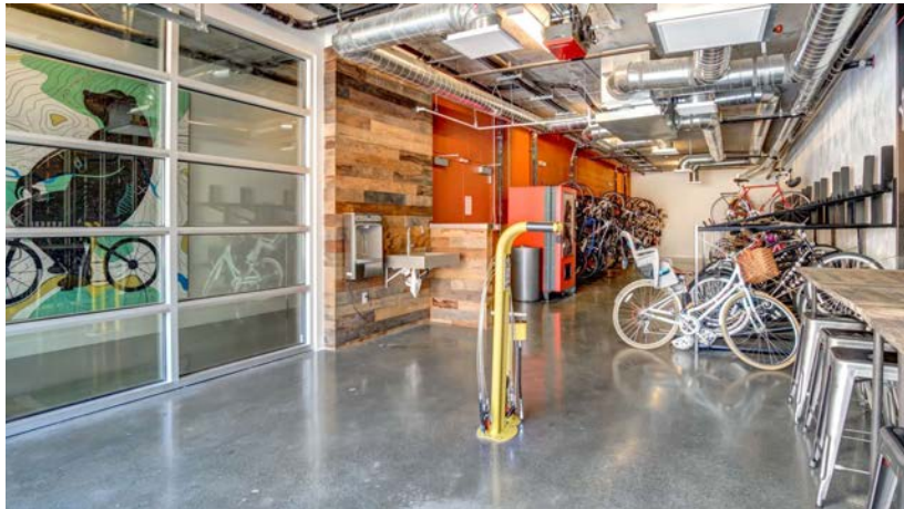
An well-equipped bicycle parking facility, located conveniently near the entry, can help encourage cycling over driving.
