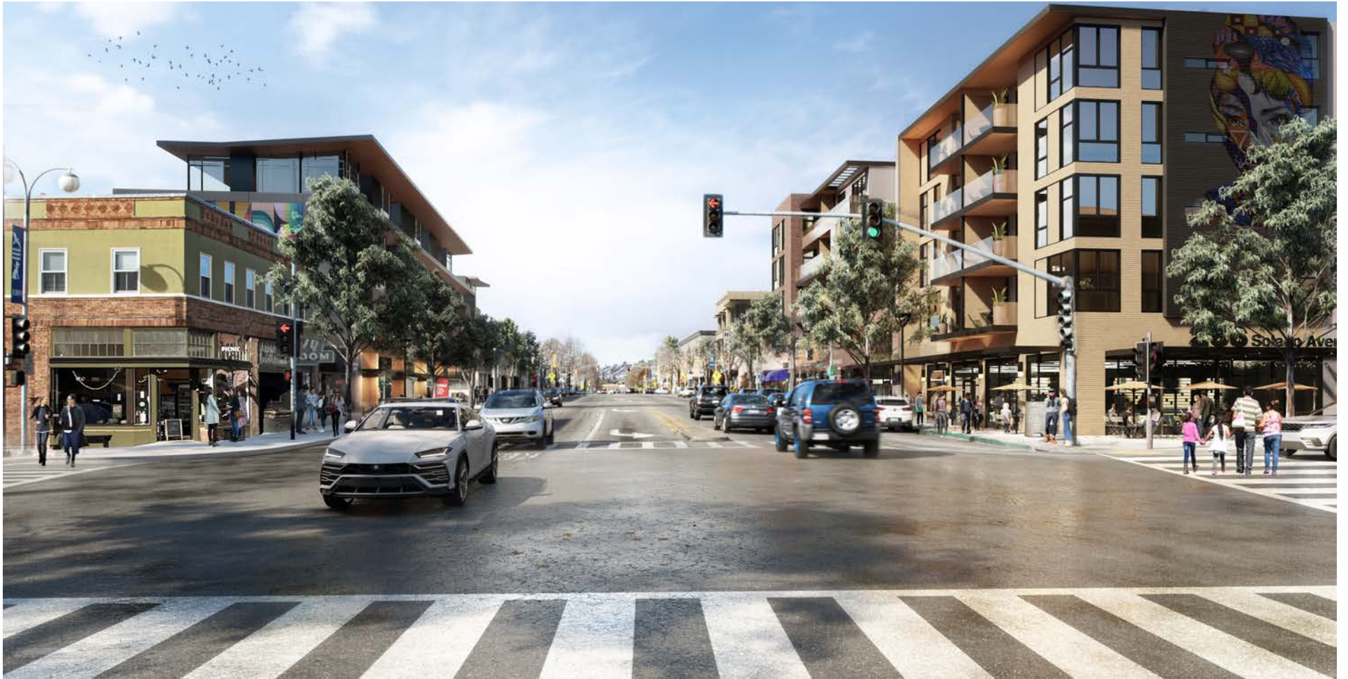
Illustration of potential future development on San Pablo Avenue looking north at the intersection with Solano Avenue
