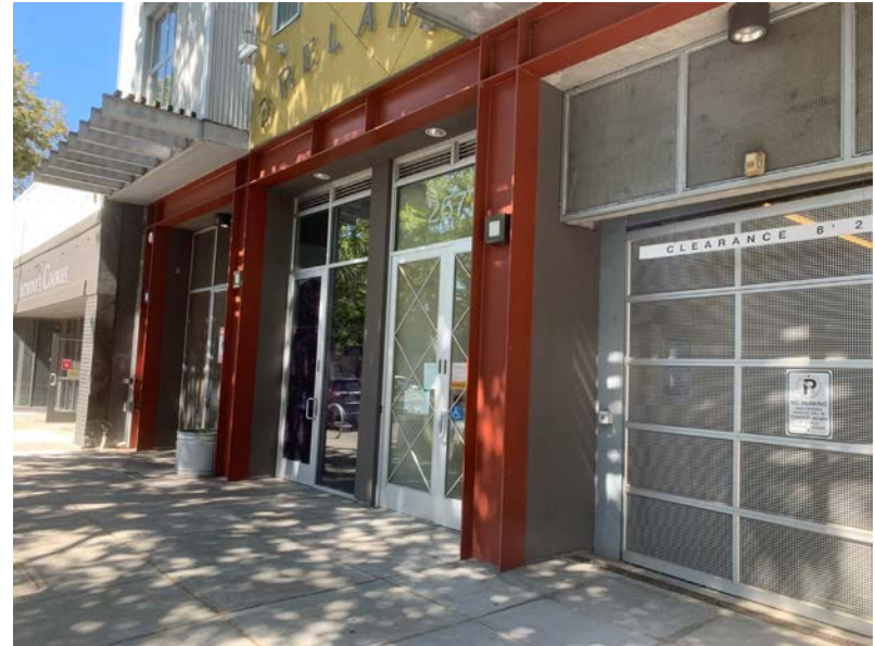
Vehicular entrances, like this one on a 50-foot wide interior lot on San Pablo Avenue in Berkeley, may be designed to be bi-directional and minimal width entrances no wider than 18 feet. The parking garage shown above is also less than 50% of the frontage on San Pablo Avenue. The parking entrance is designed so that the retail frontage and entrances are more prominent than the vehicular entrances.
