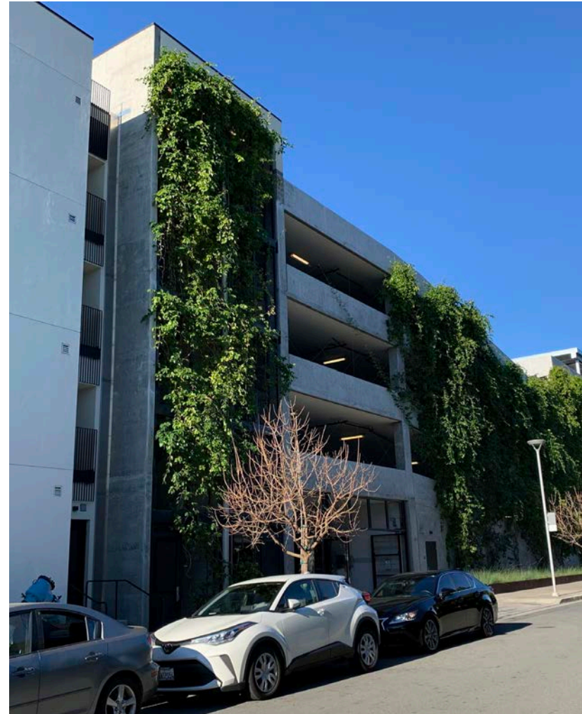
This parking garage is at the back of the site, wrapped by residential uses, except at this back edge of the property. The design uses landscaping to screen the visible portions of the parking structure.
