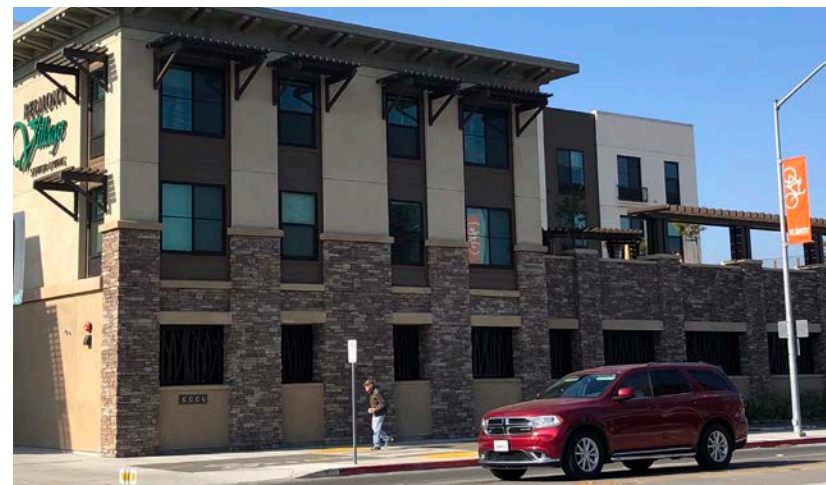
The ground level of the Belmont Village in Albany is a parking garage which is designed to be integrated with the appearance of the main building. The design includes decorative metal grates that screen the vehicles inside and human scaled, high quality materials at the pedestrian level.
