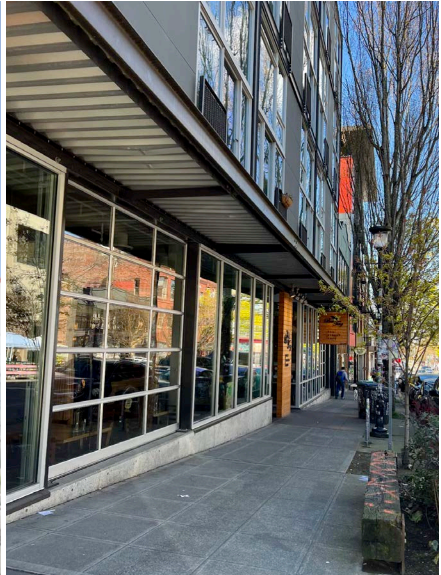
Ground-Floor commercial retail
