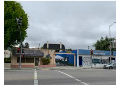
Typical Older One Story Building
