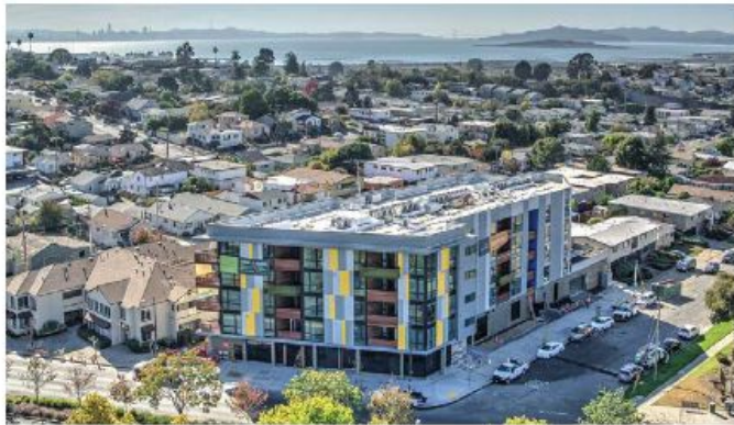
Examples of recently built multi-family housing on San Pablo Avenue in El Cerrito provide another reference for scale. Top "Credence" 10300 San Pablo Avenue, El Cerrito. Bottom: "Cerrito Vista" 10963 San Pablo Avenue, El Cerrito.
