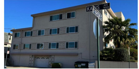
Older 4-story Apartment Building on Kains
